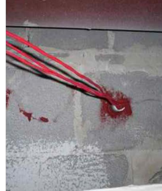
122. FIRE CAULKING NOT TO SCALE
