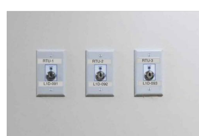
115. REMOTE TEST SWITCHES NOT TO SCALE
