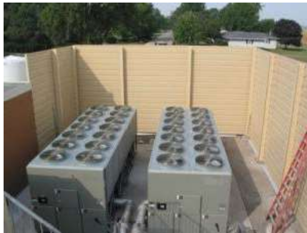
Sound Barrier Wall – Example
