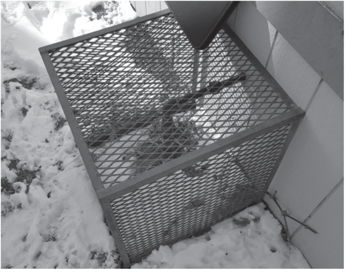
GAS PIPE PROTECTIVE CAGE
