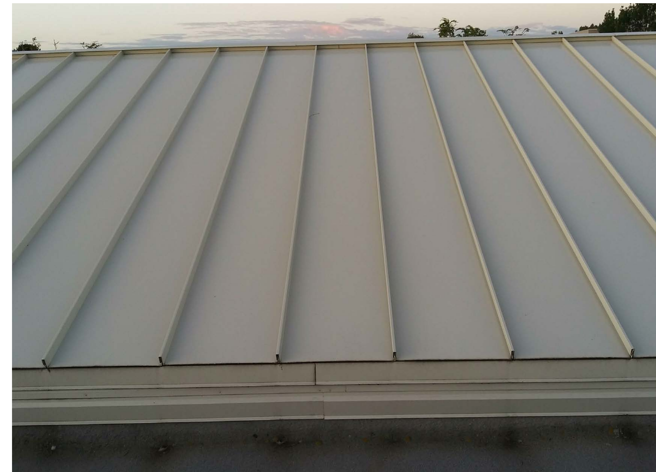
KRUSE ELEMENTARY SCHOOL - BACK OF MONITOR
