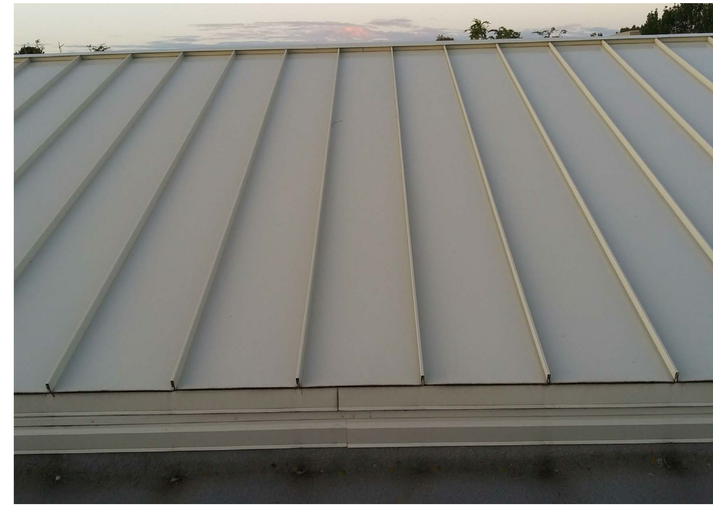
KRUSE ELEMENTARY SCHOOL - BACK OF MONITOR
