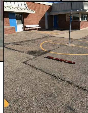
Low-lying area that is susceptible to standing water. Area should be raised during grading/paving operations
