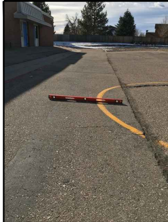
Prior to asphalt placement, underlying subgrade materials in this area should be graded to ensure water flow towards the concrete gutter.
