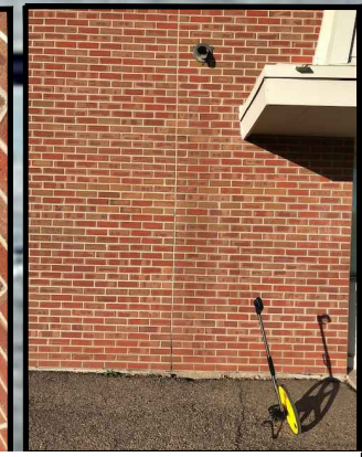
Following the placement of new asphalt, the on-set of a gap between the building and pavement should be monitored. Sealant may be required at the interface to prevent water infiltration along building.
