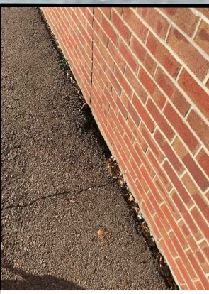
Following the placement of new asphalt, the on-set of a gap between the building and pavement should be monitored. Sealant may be required at the interface to prevent water infiltration along building.
