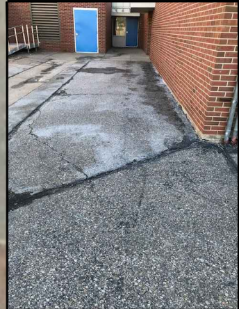
Prior to asphalt placement, underlying subgrade materials in this area should be graded to ensure water flows away from the building.
