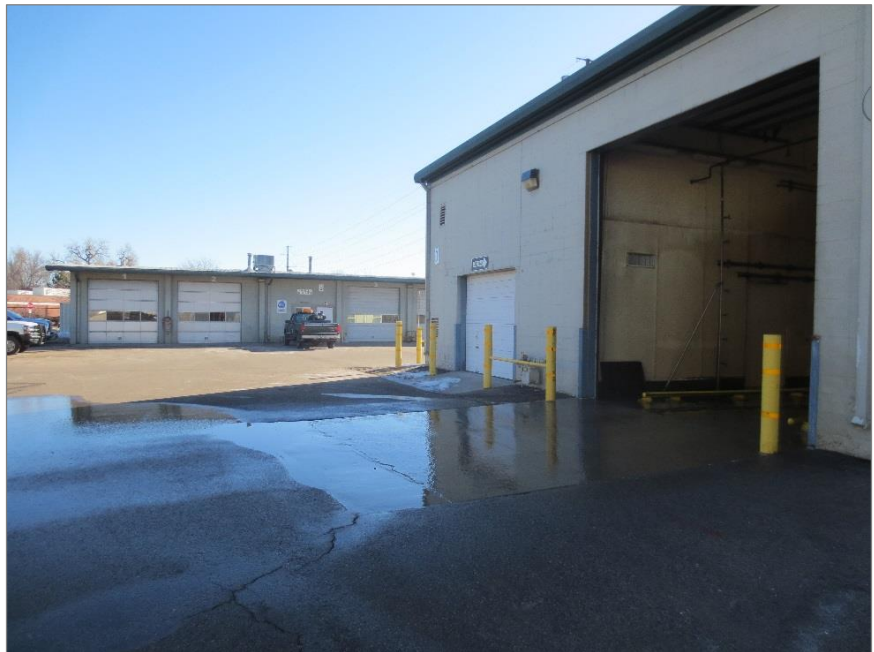
Figure 1.M - JSSC; Water running out of the Bus Wash ices during the winter and causes unsafe driving hazards.
