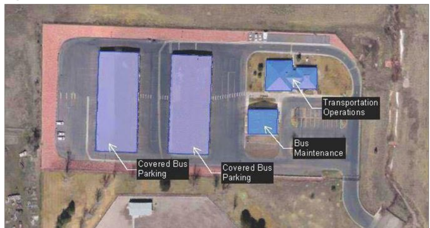
Figure 1.B - South Terminal Transportation Department
