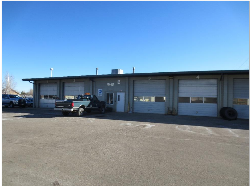
Figure 1.K - JSSC; Transportation Vehicle Maintenance Building
