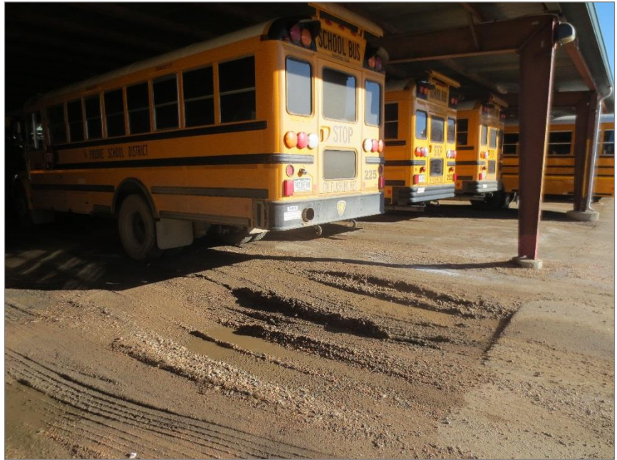
Figure 1.J - JSSC; Potholes in gravel under the Bus Canopy ice during the winter and create slipping hazards.
