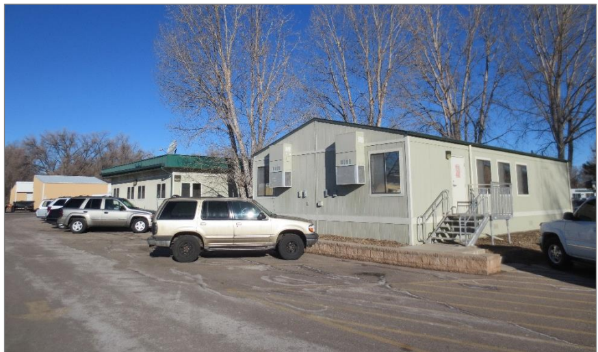
Figure 1.D - JSSC; Administration and Operations existing modular buildings.
