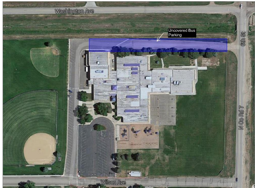
Figure 1.C - Eyestone Elementary School, Wellington, Colorado
