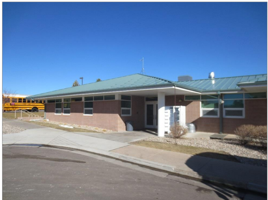
Figure 1.O - South Terminal Transportation Operations Building
