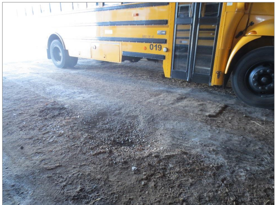
Figure 1.H - JSSC; Potholes in gravel under the Bus Canopy are unsafe conditions for Bus Drivers to walk in the dark.
