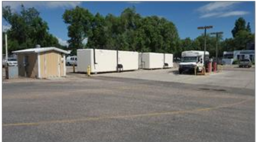
Figure 1.N - JSSC, Fuel Island at the North Terminal and main entry from La Porte Avenue
